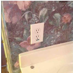
7.2.3 Outlet is not on a GFCI protected circuit. This needs to be corrected for safety. (Garage)
